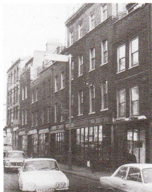
The Comyn Ching Triangle (Monmouth/Mercer/Shelton Streets) – viewed from Monmouth Street in 1974 – has been largely restored to provide housing, shops and offices with an internal courtyard.
