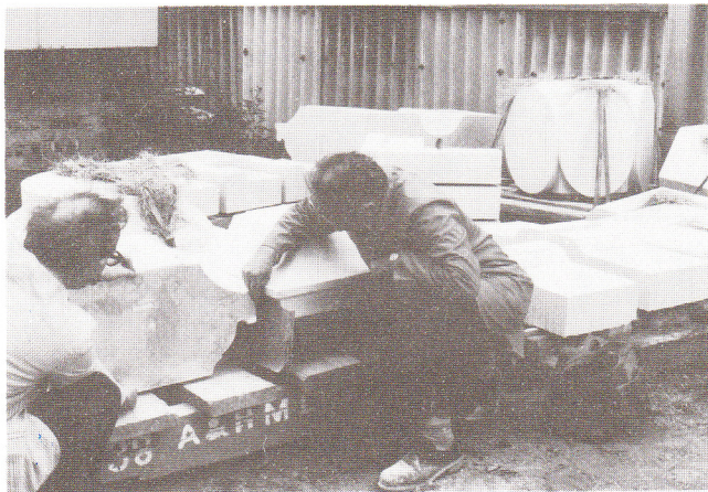
Architect 'Red' Mason and Works Supervisor Alan Watts, at Ashby & Horner Stonemasonry, checking the cornice to the pedestal against the zinc template.
