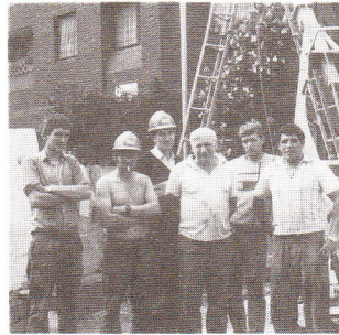
The Foundation Site Team are pictured in front of the Piling Rig with the Tunnelling Team on the left and the Piling Team on the right.
