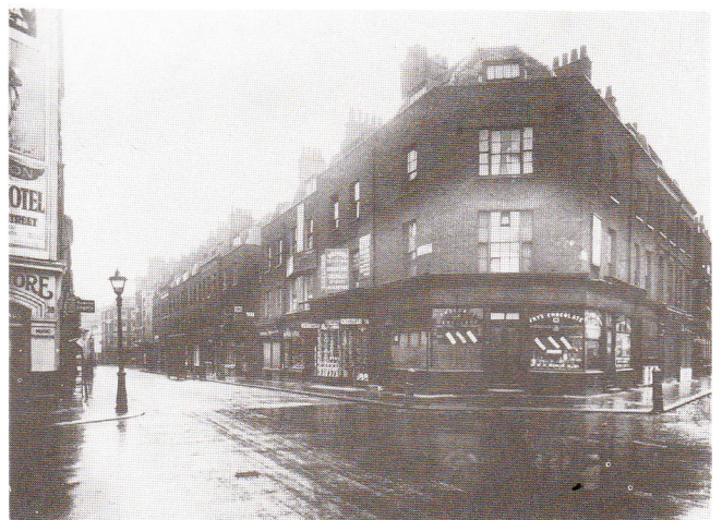
Photograph c1900 showing Monmouth Street (south) and Earlam Street. The Monument Committee has pressed for the removal of the petrol station now occupying this site so as to completely re-instate Seven Dials. The site is now being redeveloped.
